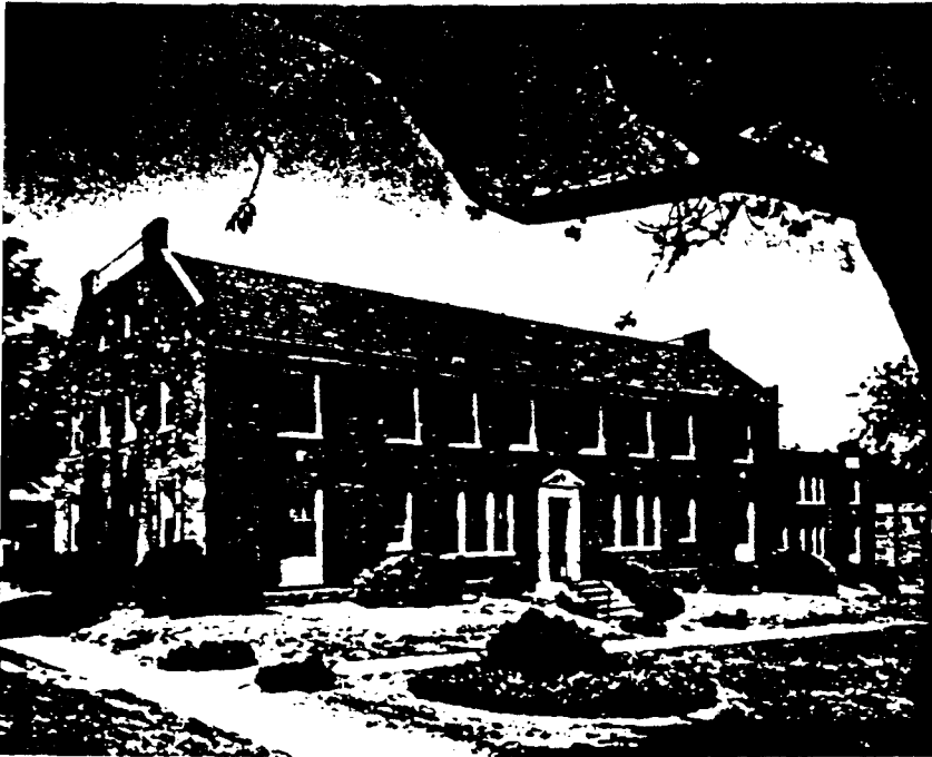
One of the many varying designs of the Colonial Revival buildings that form the garden apartment complex of Colonial Village.
